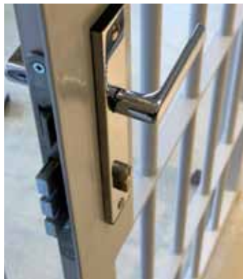
Detail of the multilock in operable bars
