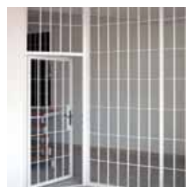
The whole entrance is protected by a grillage wall
