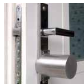
Electromotor manipulation of the safe locking mechanism of the door
