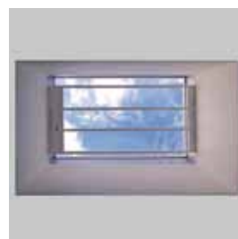
Lockable swing-away bars for a small window
